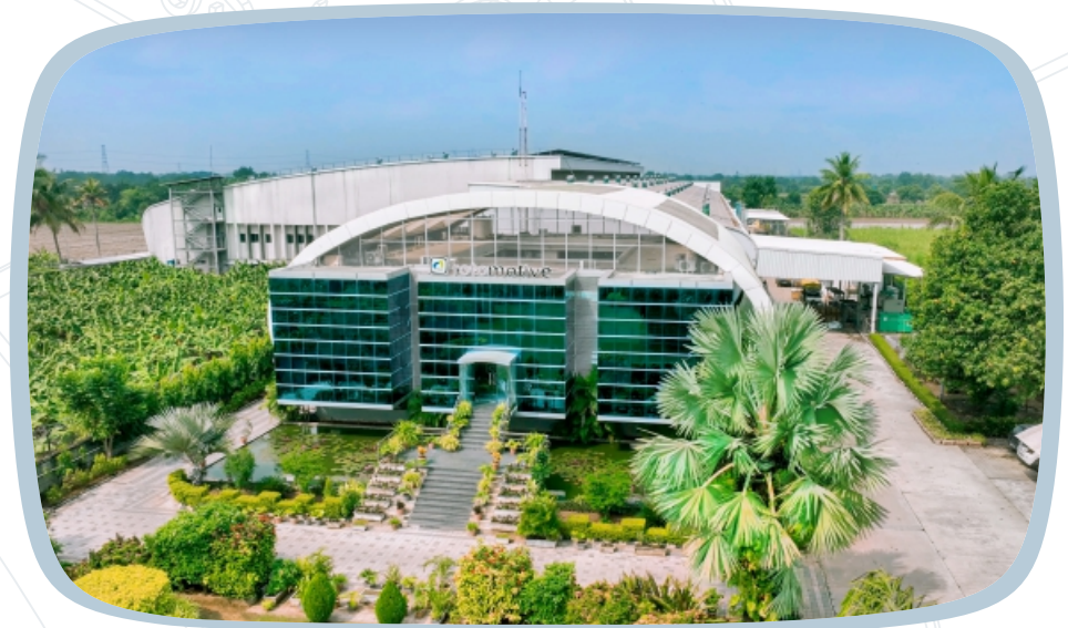
Motor manufacturing facility, India
