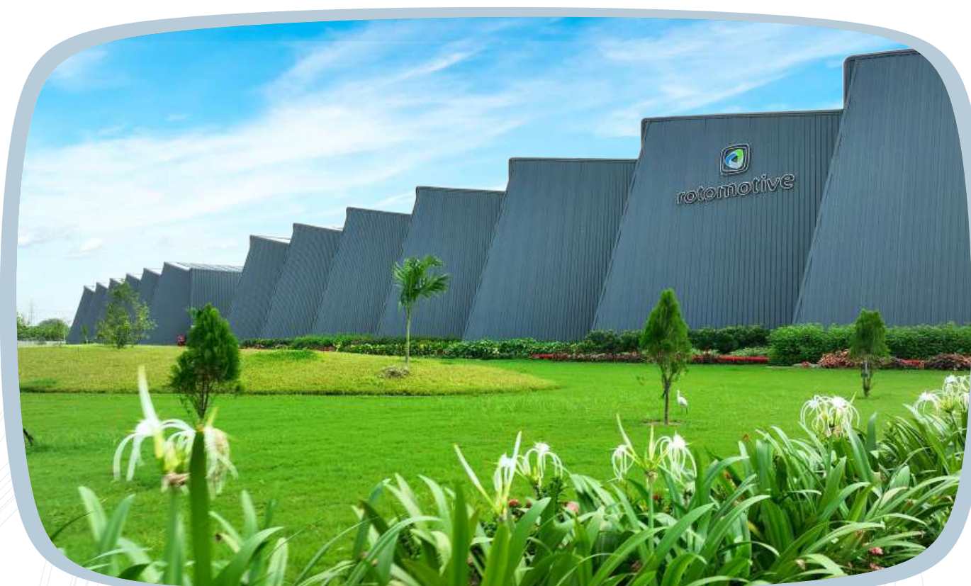
Gearbox Manufacturing Facility, India
